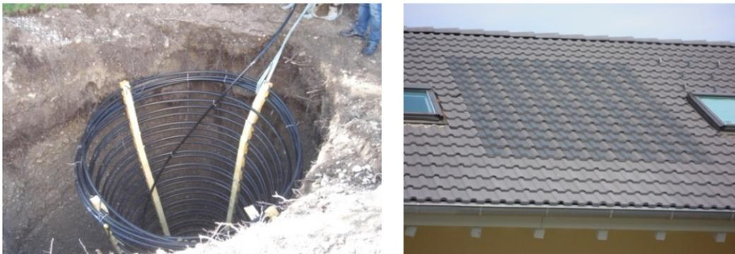
Fig. 2. (a) Geothermal energy baskets, (b) solar roof tiles [Pictures: A. Drexler, A. Loose]
