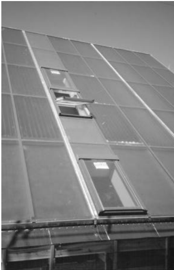
Abb. 2: Solar Roof in Rostock-Brinkmanshöhe (Fa. Solvis, Architekt: Carewicz, AP, Rostock)
