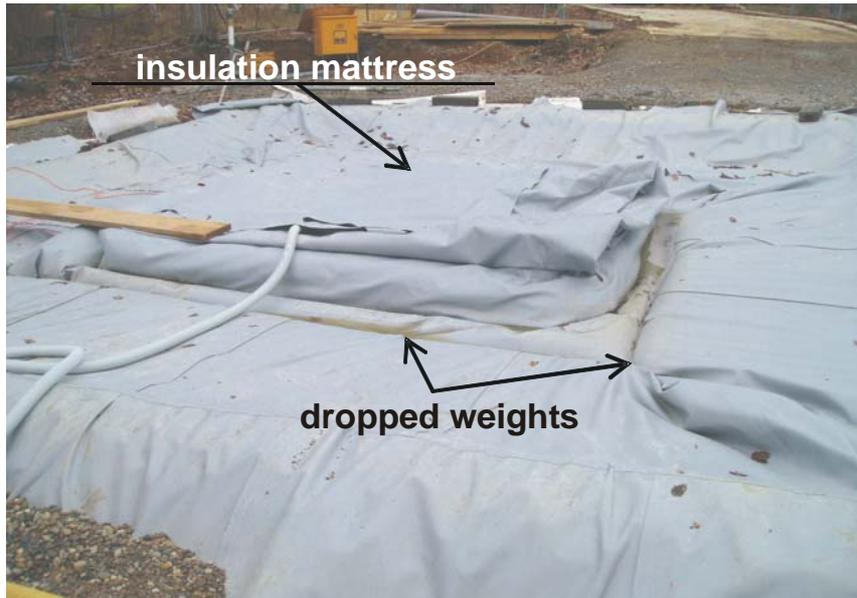
Figure 5: Photo of the floating cover, edges area not yet insulated
