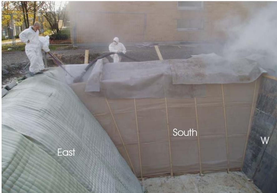
Figure 2: Air injection of the insulation (foam glass granules) from the silo-truck, and from left to right: geocontainer, membrane formwork and prefabricated wooden formwork.
