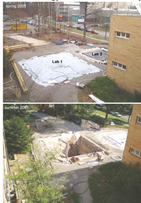
Figure 1: Outdoor laboratory: research store at ITW; top laboratory 1: hot-water pit heat store with floating cover, laboratory 2: gravel-water-store; bottom laboratory 1 after deconstruction
