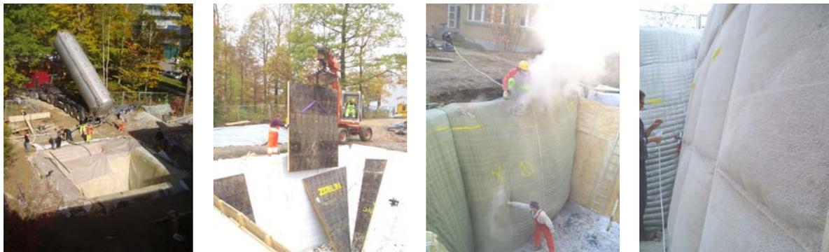
Figure 2: Construction methods for the installation of bulk thermal insulation in lost formwork. From left to right: installation of the insulation by blowing from a silo-truck (air injection), mounting prefabricated formwork elements, geotextile during filling and (jute-) membrane formwork (compare Ochs 2005a)
