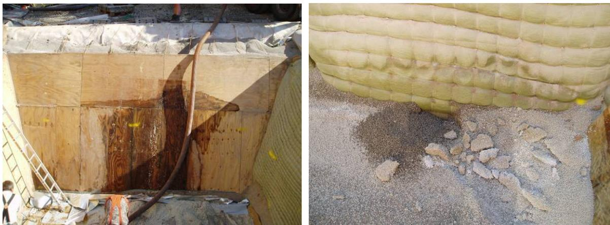
Figure 6: Moisture penetration of the north slope (L1 W4) and the bottom insulation (L1 B) after the deconstruction of the research store
