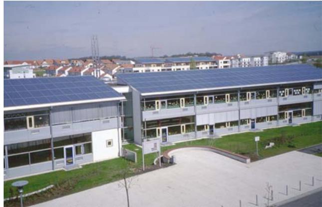
*Figure 4: Solar collectors installed on the roof of a school in Neckarsulm*
