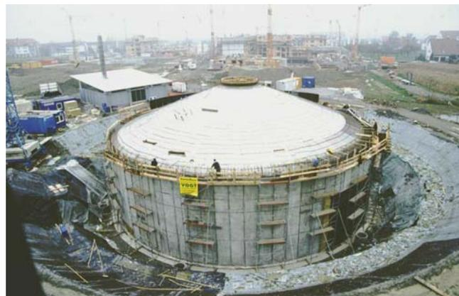
Figure 3: Hot-water heat store in Friedrichshafen during construction
