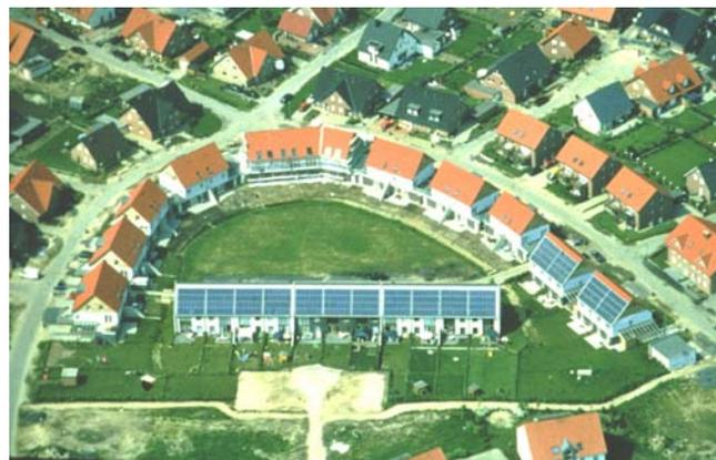
*Figure 6: Solar assisted district heating system in Steinfurt-Borghorst*
